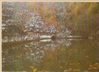
Barajul microhidrocentralei Petros The dam of Petros micro-hydroelectric plant
